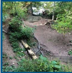
CONCENTRATED RUNOFF Some locations with concentrated runoff from adjacent properties are causing erosion and damage to retaining walls
