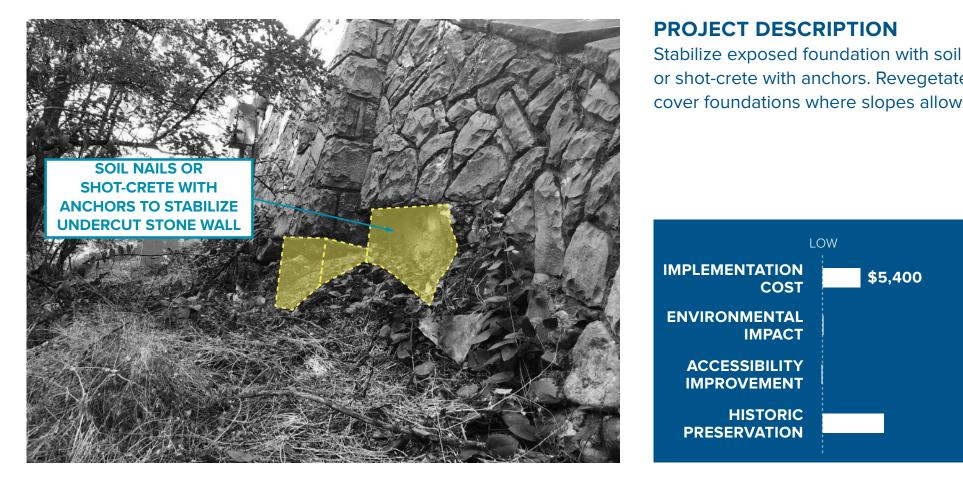
**PROJECT DESCRIPTION** Stabilize exposed foundation with soil nails or shot-crete with anchors. Revegetate and
