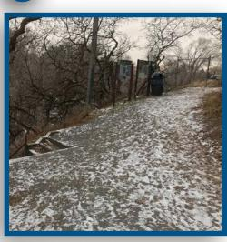
STEEP CROSS SLOPES Some segments of the trail have steep cross slopes (higher than 2%) that limit the accessibility of the park.
